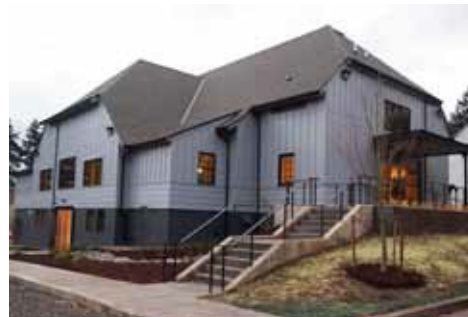
American Legion Hall after renovation
