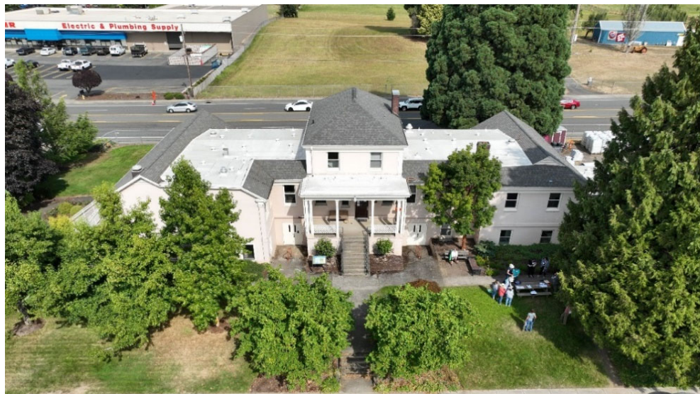
78th Street Heritage Farm Administration Building
