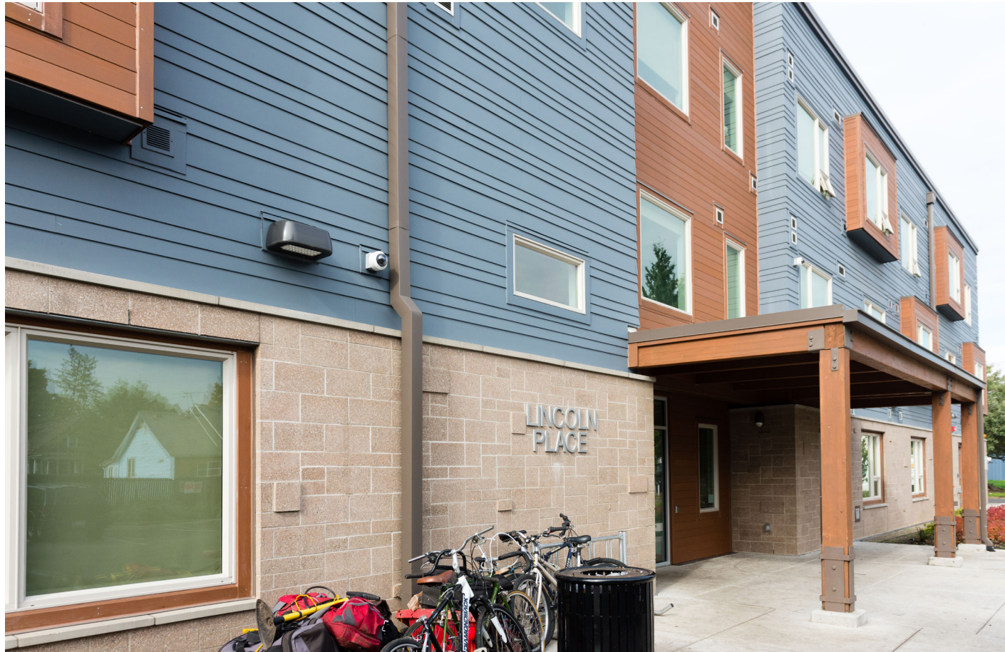
In designing Lincoln Place, local leaders toured supportive housing buildings in Seattle and Portland and used a similar design.
