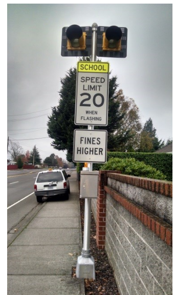
School Speed Limit Flashing Beacon
