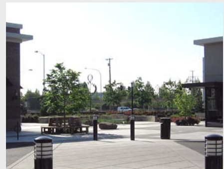
Figure 5-39. An example of a walkway with bollards that include light fixtures to clearly define the pedestrian access where it crosses a driveway (Clark County).
