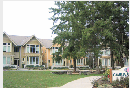
Figure 5-27. Common open space example (Bainbridge Island, WA).
