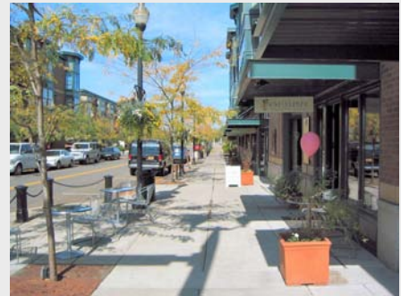
Figure 5-17. Widened sidewalk area may be used to comply with pedestrian-oriented space standards (Orenco Station, OR).
