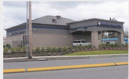
Figure 5-60. The landscaping in front of the Riverview Bank's drive through meets the intent of the standards and the canopy certainly adds visual interest. However, more windows would be needed on the façade to comply with transparency requirements herein (15% would be required for this property, within the Transitional Overlay).
