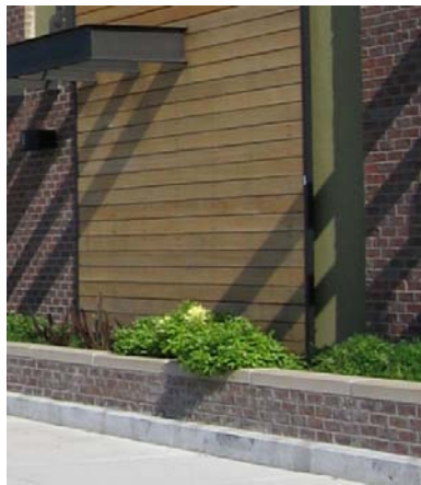
Figure 5-40. Elevated planter between a walkway and building (Vancouver, WA).
