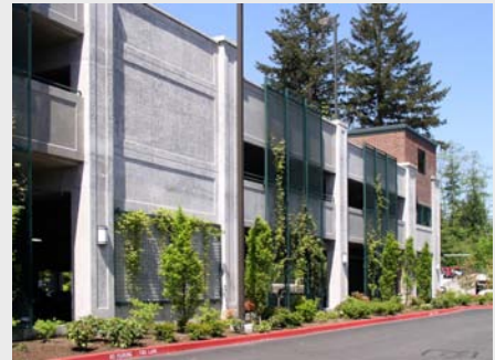
Figure 5-62. The trellis and vines, landscaping, and facade design is a good example of design treatments for garages visible from an internal access road (Mill Creek, WA).
