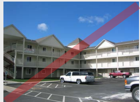
Figure 6-13. Roofline modulation alone does not help this building to meet articulation standards.
