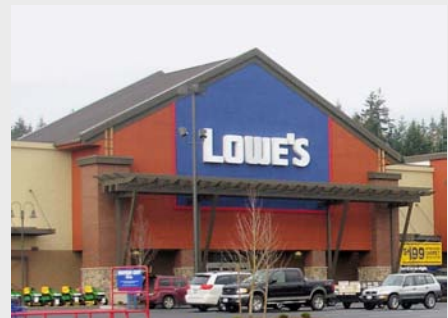
Figure 6-19. This building has a simple, prominent entryway with a pitched roof, and distinctive use of materials and colors (Monroe, WA).
