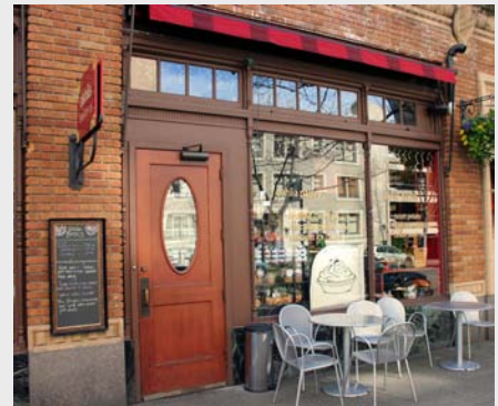
Figure 6-29. This façade uses a decorative door, windows, materials, blade sign and a retractable awning (Seattle, WA).
