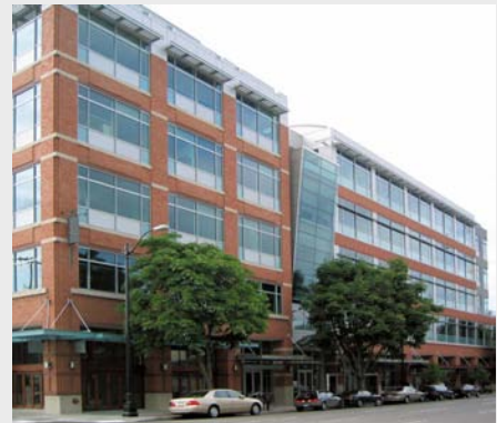
Figure 6-22. The leaning glass wall in the middle of the upper floors effectively breaks up the massing of this façade (Seattle, WA).
