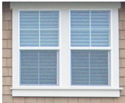
Figure 6-38. An example of trimmed windows.
