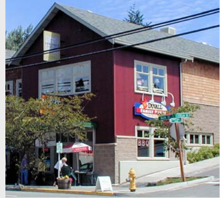
Figure 6-40. This building uses an acceptable combination of metal siding, concrete block and wood shingles (Duvall, WA).
