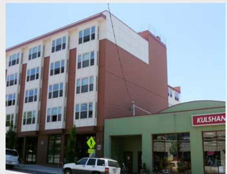
Figure 6-49. Acceptable fire wall design.
