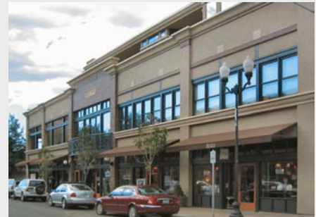
Figure 6-3. This building uses distinct window patterns, vertical piers, and separate awnings to articulate the façade (Bend, OR).
