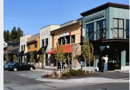
Figure 6-4. This building is designed to look like several small buildings, each with a distinct façade (Juanita, Kirkland, WA)
