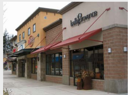
Figure 6-43. This building combines stucco and concrete block.
