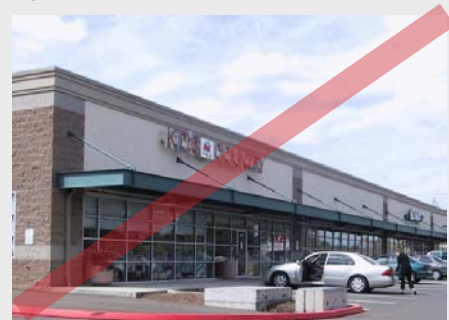
Figure 6-5. No substantial façade articulations.
