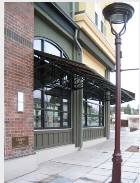
Figure 6-27. This building uses decorative materials, windows, lighting, and canopies. The Year of Construction plaque is also a nice detail (Juanita, Kirkland, WA).
