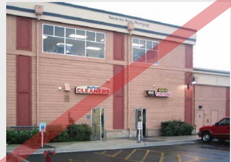
Figure 6-36. Weather protection would improve this secondary entrance.
