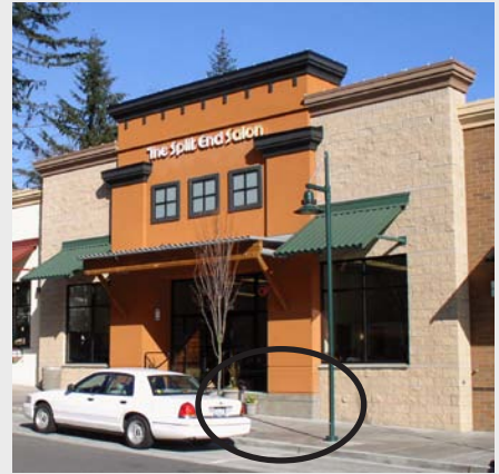
Figure 6-44. Acceptable use of stucco and concrete block. Note how concrete base is used for stucco portions of the façade (Mill Creek, WA).
