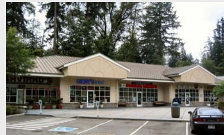
Figure 6-8. The change in roofline combined with the vertical modulation along the façade make this an acceptable design (Bellevue, WA).
