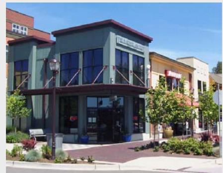
Figure 6-56. A turret-like feature with corner canopy and cropped entry (Kirkland, WA).
