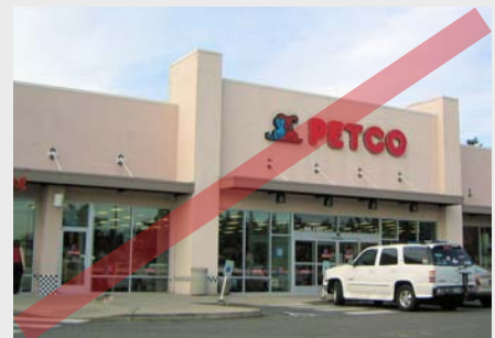
Figure 6-30. The tile work would marginally qualify as a detail, but the simple wood canopy would not and no other features here would qualify as a detail.
