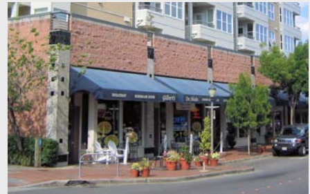
Figure 6-41. An example of an acceptable mix of smooth and split-faced concrete blocks (Bellevue, WA).
