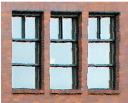
Figure 6-37. An example of recessed windows.
