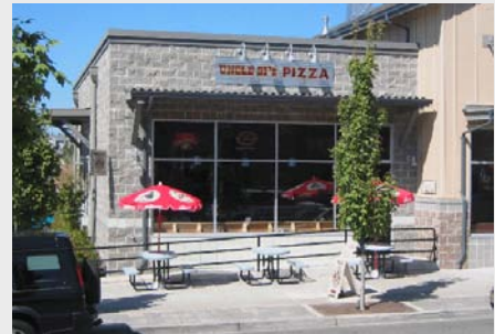
Figure 6-42. This building employs a single type of concrete block, but it comprises less than 50% of the façade (Snoqualmie, WA).
