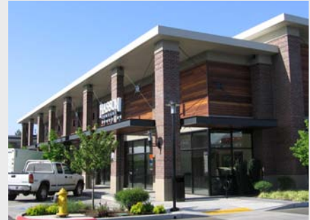
Figure 6-25. This building uses a decorative arcade, steel canopies, custom light fixtures, and a distinctive mix of materials. (Vancouver, WA)
