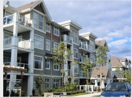
Figure 6-11. This building uses projecting balconies, roofline modulation, and repeating window patterns (White Rock, BC).
