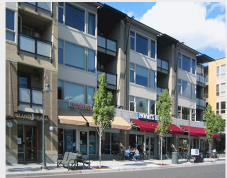
Figure 6-12. This building uses vertical building modulation (recessed balconies), repeating windows, and a distinctive top/middle/bottom (Mercer Island, WA).
