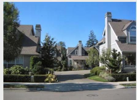
Figure 7-55. Homes configured around a shared, paved courtyard (Issaquah Highlands, WA).
