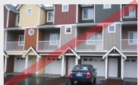
Figure 7-18. Bad: Individual private driveways from a street; no landscaping.
