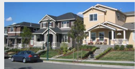
Figure 7-43. Garages in rear off an alley (Issaquah Highlands, WA)
