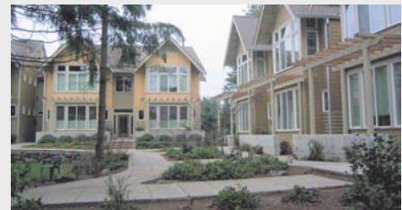
Figure 7-10. Two-story units surrounding a shared garden courtyard (Bainbridge Island, WA).
