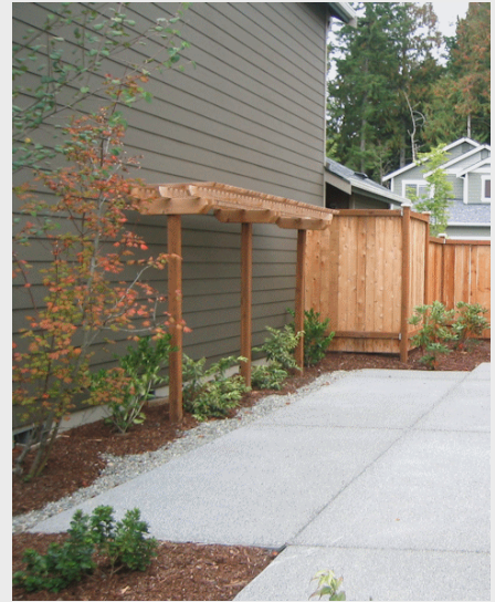
Figure 7-48. Side yard and privacy wall example, in a zero lot-line configuration (Lacey, WA).
