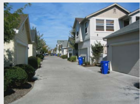
Figure 7-58. ADU built over a garage off an alley (Orencia Station, OR).
