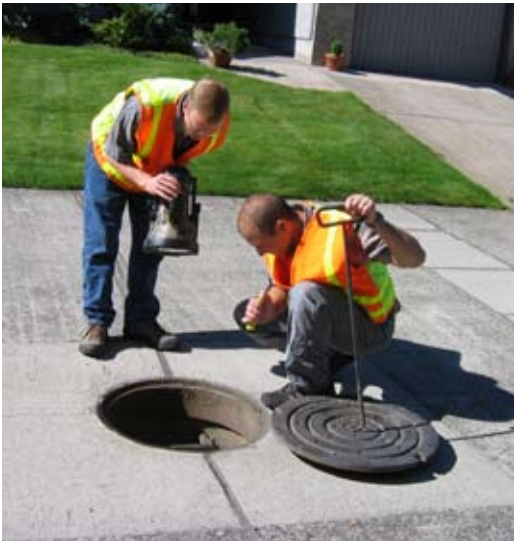
Program staff check for signs of illicit discharges to the stormwater system.
