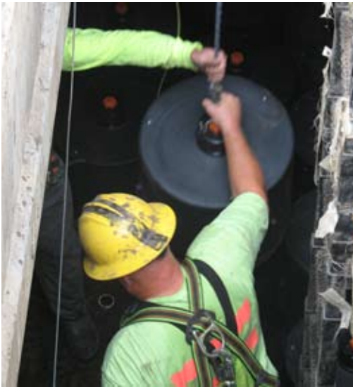
Crews replace stormwater filter cartridges.
