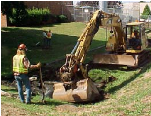
Maintenance crews repair a bioswale.
