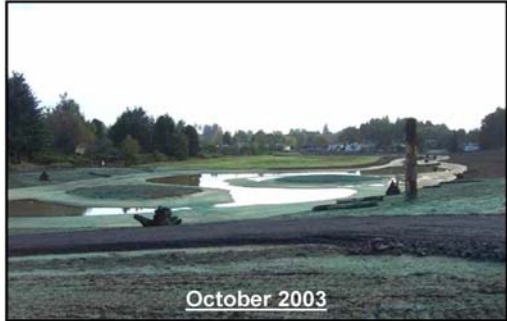
Shortly after construction and hydroseeding.
