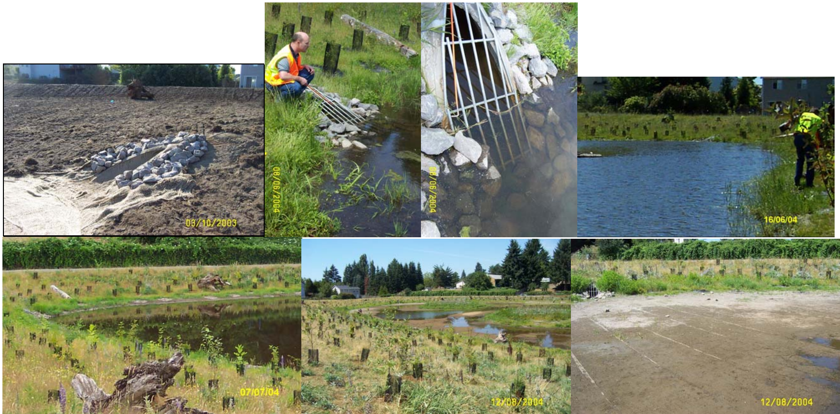
Figure 6 Thomas Wetland Outflow After Construction and Summer 2004 Drop in Water Surface.
