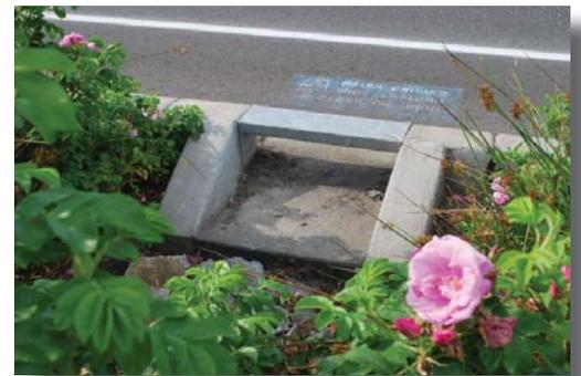
Water flowing off impervious surfaces (for example a roof or driveway) can be delivered to the rain garden through a swale lined with decorative rock or plants, through a pipe, or across a landscape area.
