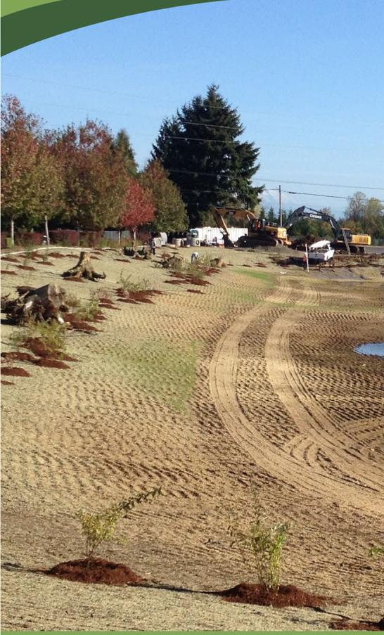
The Clean Water Program has recently partnered with Clark County Public Works to construct a new stormwater pond in the Curtin Creek watershed. The project created a 4.0 acre stormwater pond that will hold 2.3 million gallons of runoff or enough to fill a football field 5 feet deep! The pond will collect and treat runoff near the intersection of the Padden Parkway and Andresen Road (from current pavement, as well as future anticipated expansion of the intersection).
