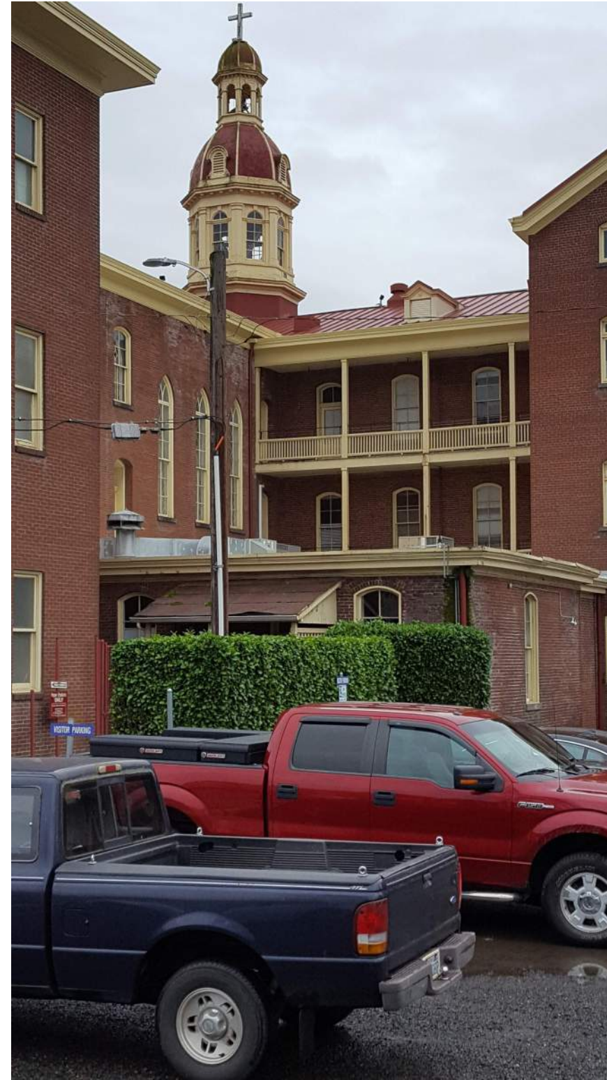
AFTER REPLACING DORMER WINDOW WITH LV-5
