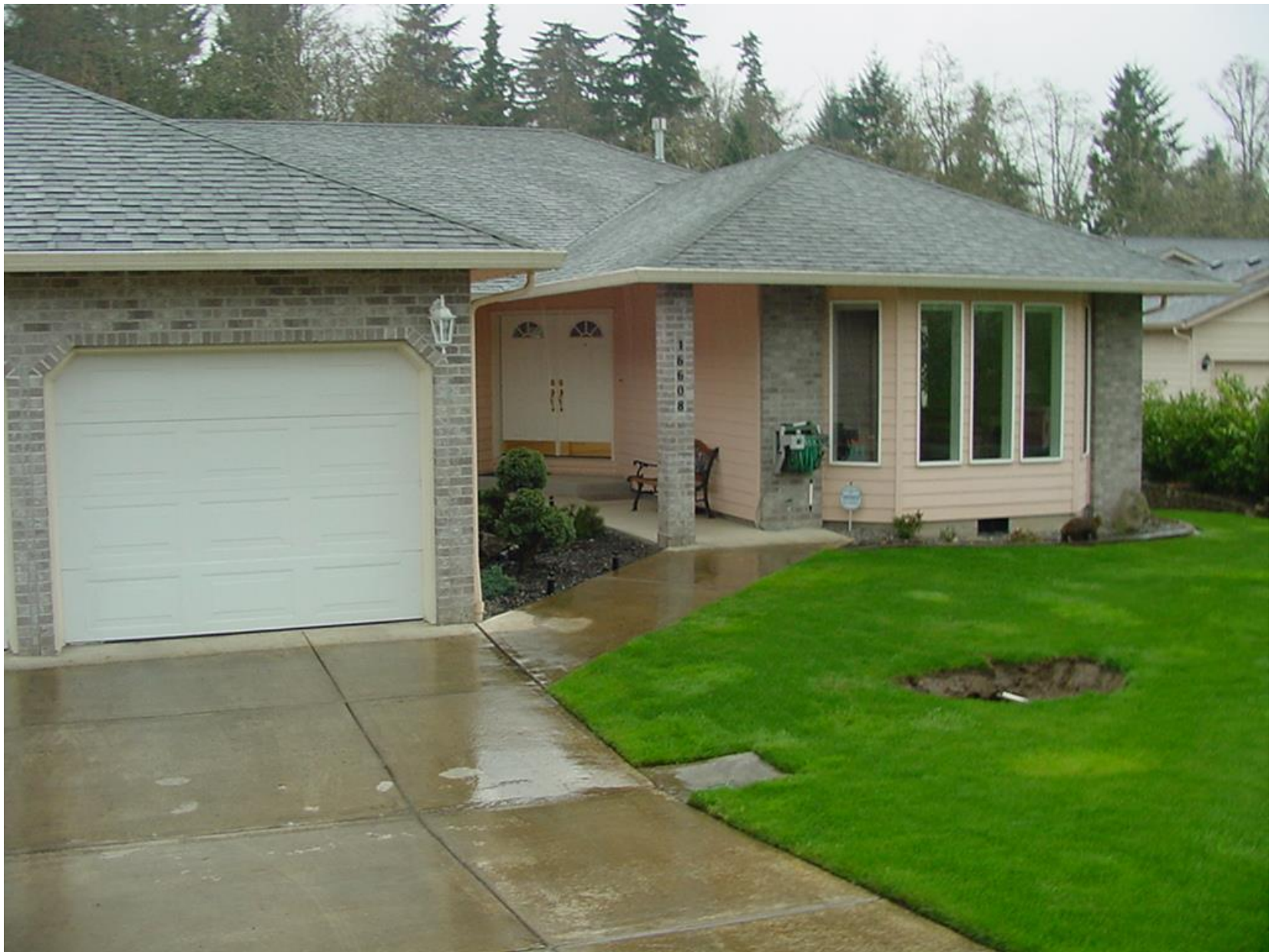
This sink-hole showed up in 2001--the ground just started slowly sinking; you could actually hear water running very deep in the hole.
