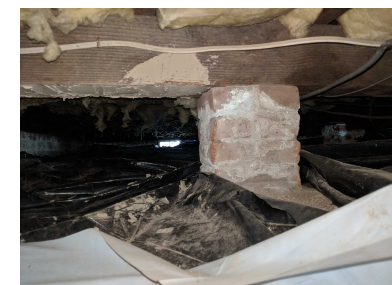
B PHOTO - TYPICAL BRICK PIER
