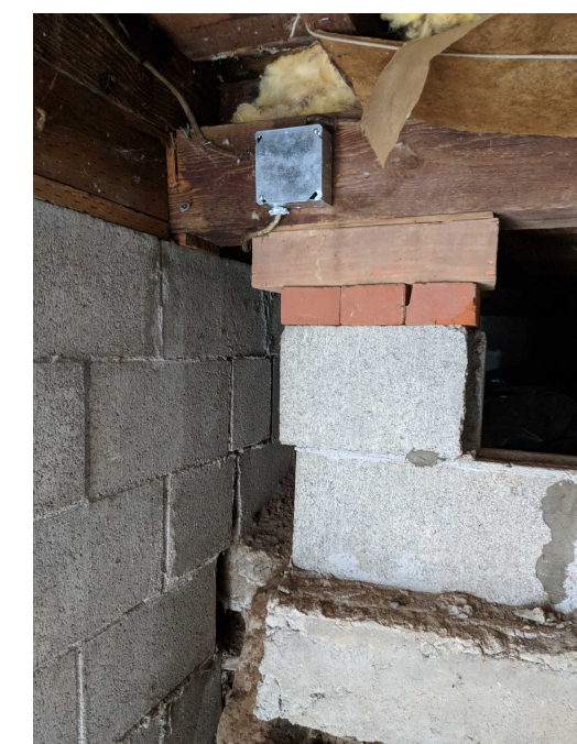
C PHOTO - EXISTING BEAM SUPPORT
