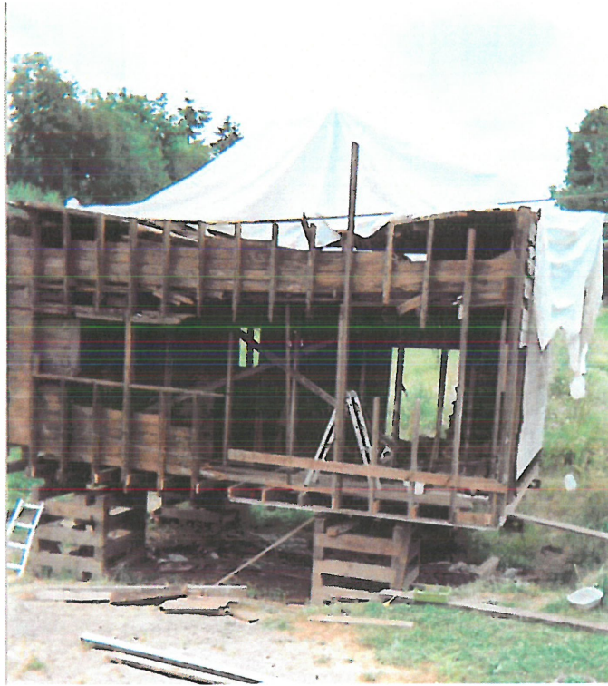
Granary on blocking, new floor joists installed, west wall siding removed beginning to replace rotten studs
