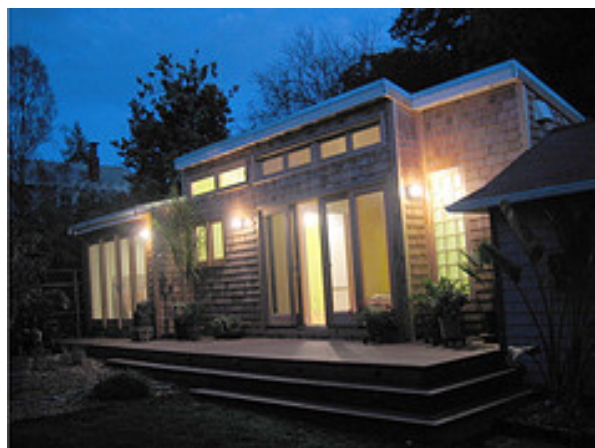
This backyard Accessory Dwelling Unit (ADU) in the San Francisco Bay area has a living room, bedroom, kitchenette and bath, all in about 400 sq. ft.
