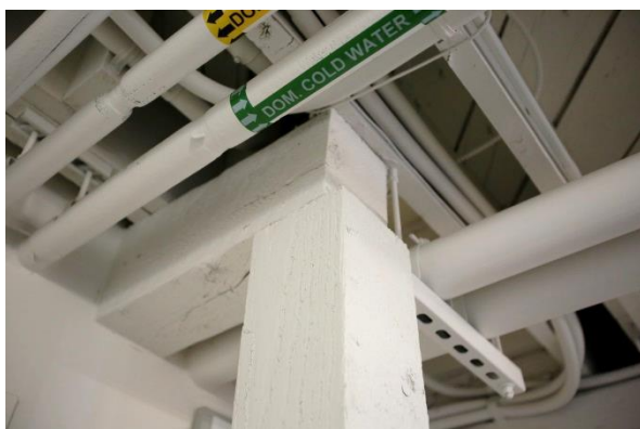
Unattached post-and-beam frame
