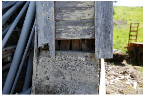
Rotting wood framing member
