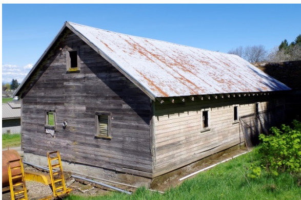
Rusted metal roof
