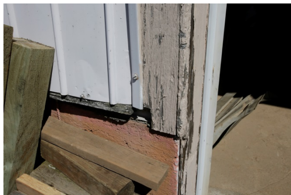
Deteriorated wood and peeling paint
