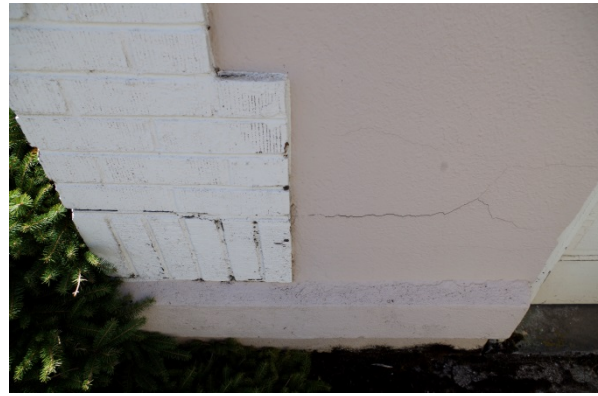
Structural cracking at the northeast corner
