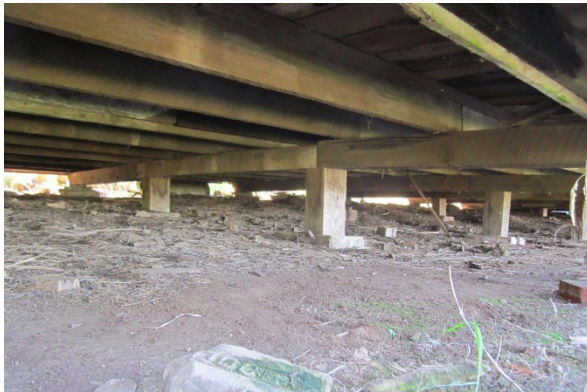
Bowing foundation beams
