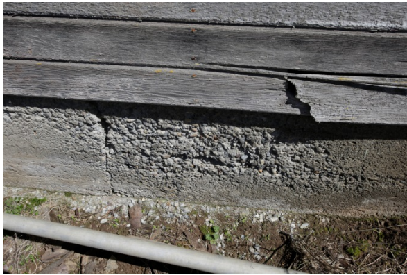
Spalling foundation
