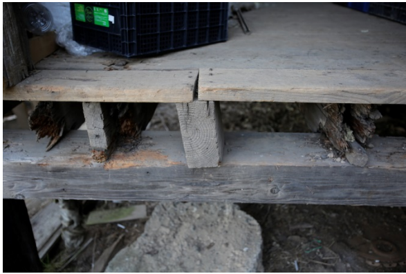
Rotting floor joists
