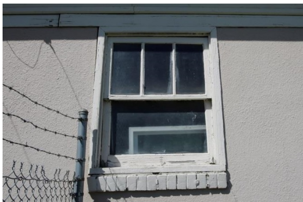
Broken window frame
