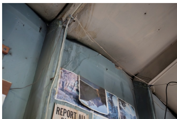
Warped and stained interior wall panels
