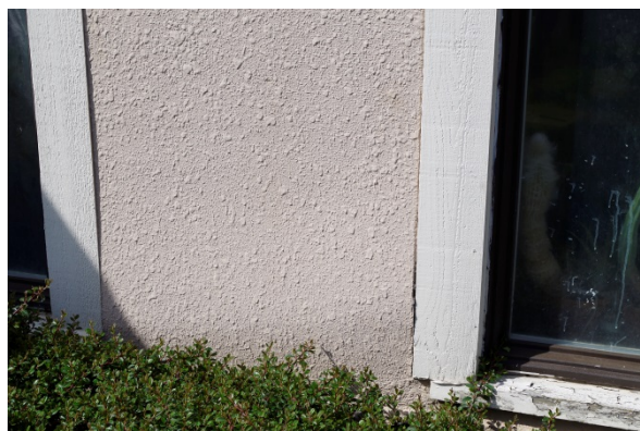
Warped insulated paneling on the south wing
