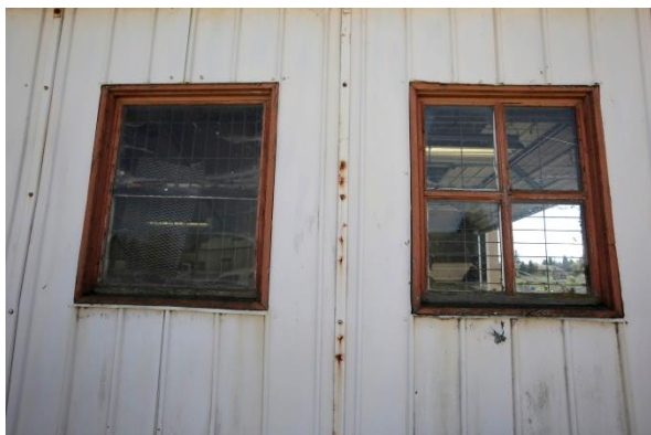
Rotting wood window frames
