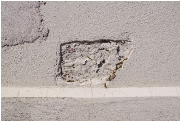
Exposed structural block on south elevation
