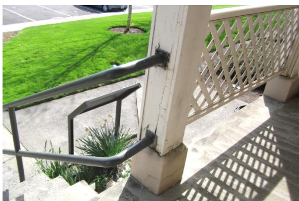
Peeling paint on south porch column
