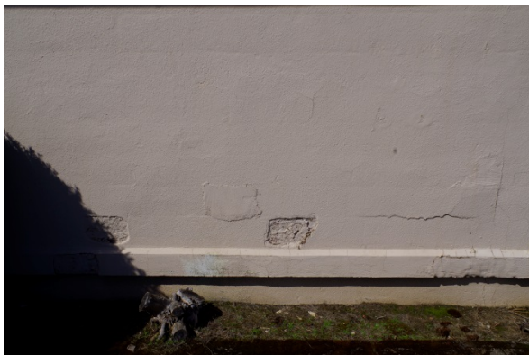
Exterior stucco cracks
