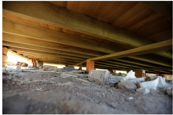
Sagging foundation beams
