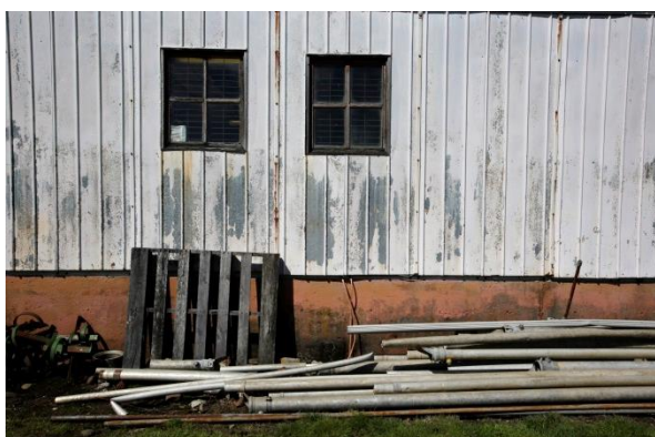
Rusting metal siding and peeling paint
