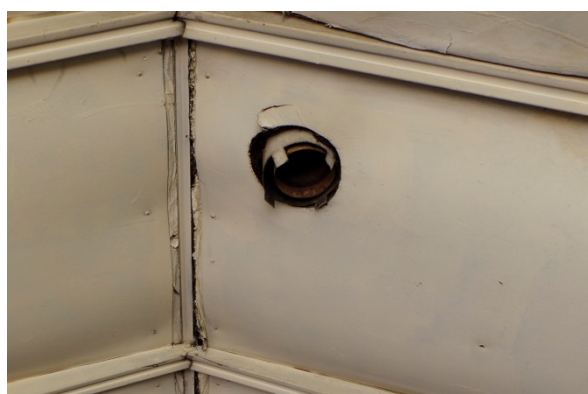
Abandoned chimney openings
