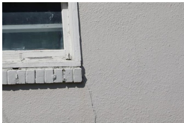
Structural cracking on south elevation
