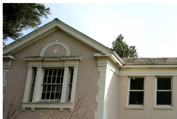
Broken cornice on north façade
