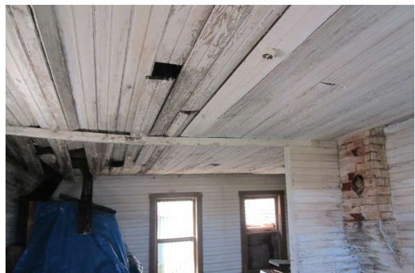
Collapsing ceiling
