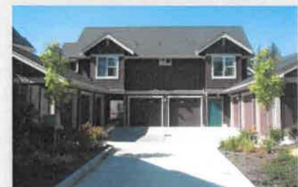
Figure 9-27. Example of accessory dwelling units built over garages for cottage development (Issaquah, WA).
