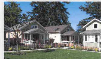
Figure 9-26. Greenwood cottages (Seattle, WA).
