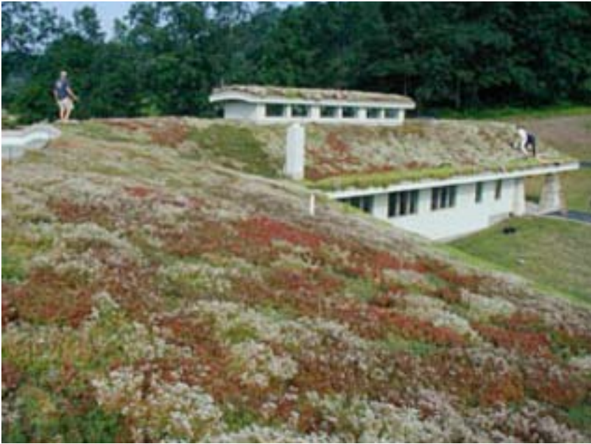
■ FIGURE 4-5. Green Roof
