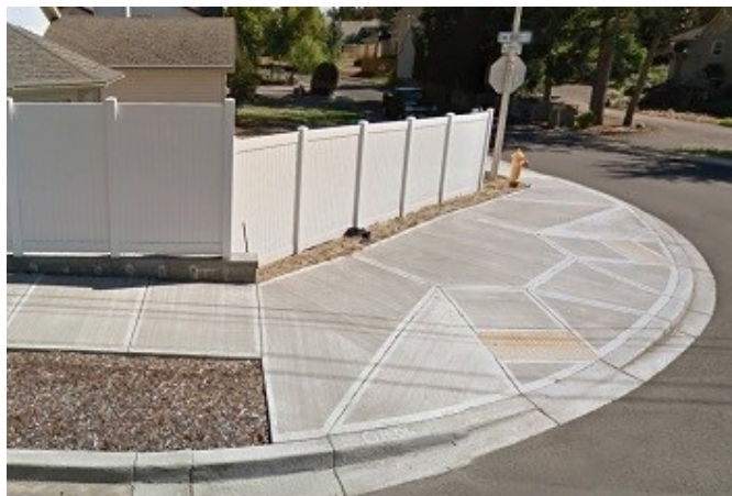
A street corner with disabled-accessible sidewalk curb ramps.
