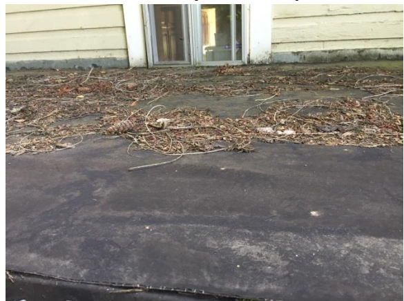
Exhibit 3 Roof Showing Membrane Lifting
