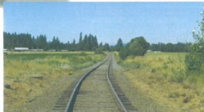
View near MP-8.7. Narrow 60-foot ROW and potential rail operations conflicts in area proposed for rezoning to Railroad industrial will require coordination of trail alignment with development code and site design to maintain trail continuity.
