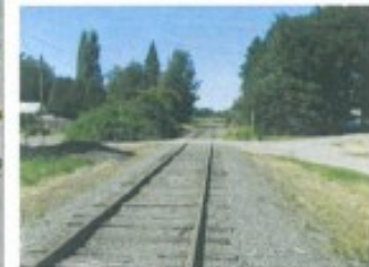
Driveway crossing north of NE Laurin Road near MP-8.5. The recommended alignment is left of track.
